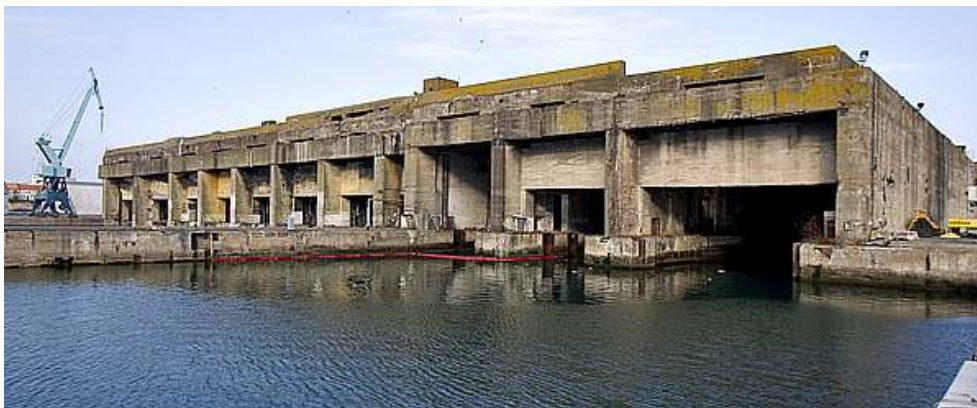
Fig. 1. Submarine base (WWII) of the port of La Pallice seen from the southwest
